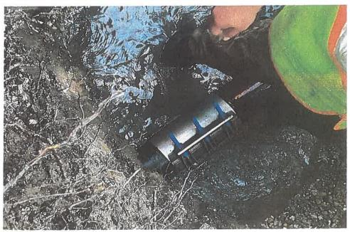
(Above): A 12" repair clamp used to fix the 6" water main.
